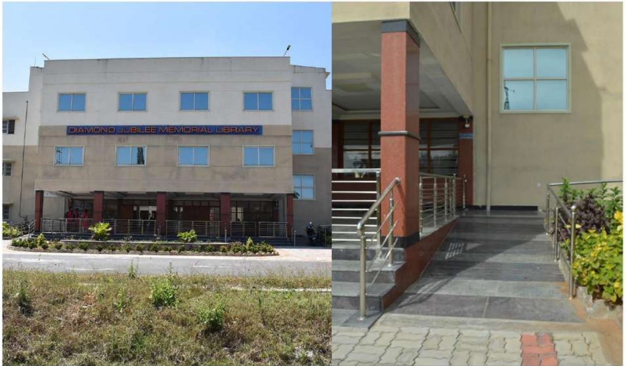
Elevator and Ramp facility available in the Library Block
