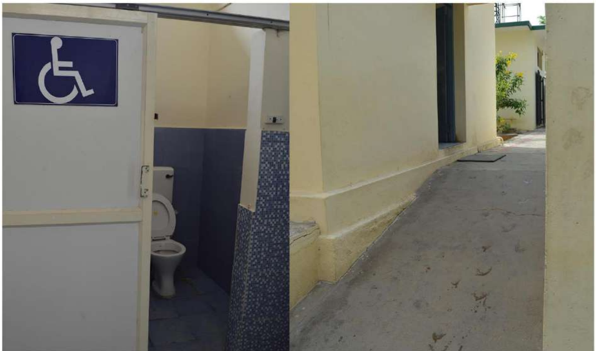
Special lavatory facility available for Students with disabilities
