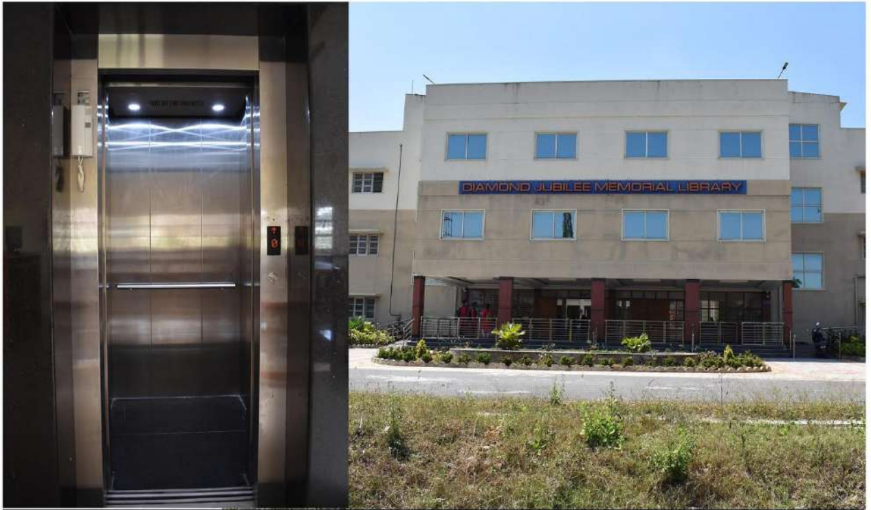
Elevator facility available at the Library Block
