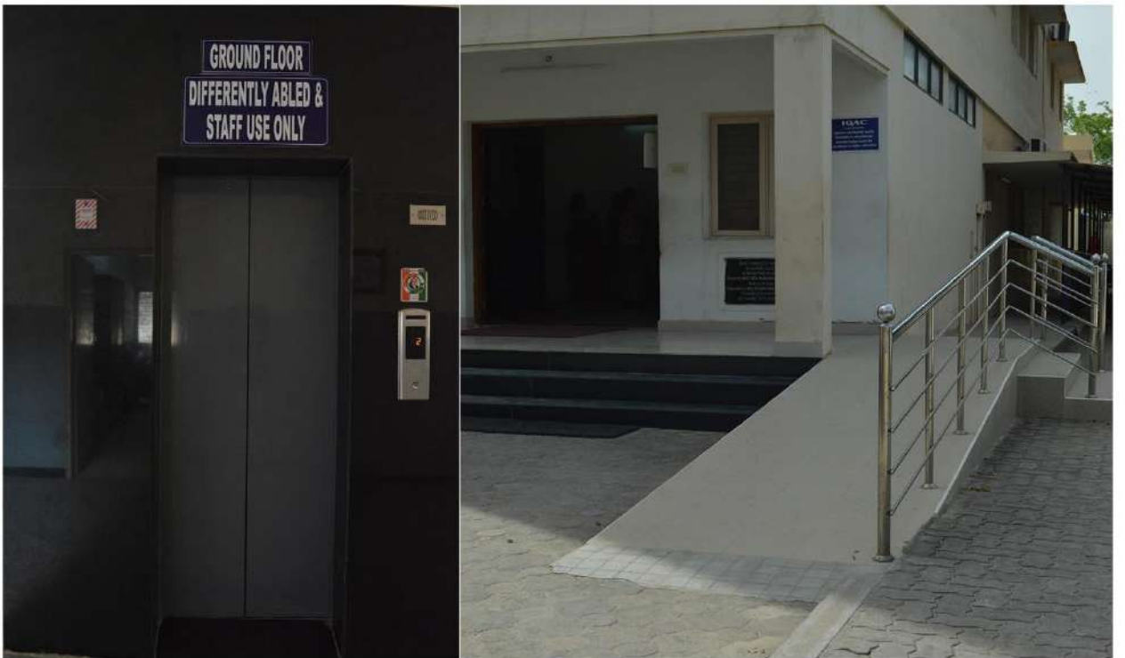
Elevator and Ramp facilities available at the Admin Block
